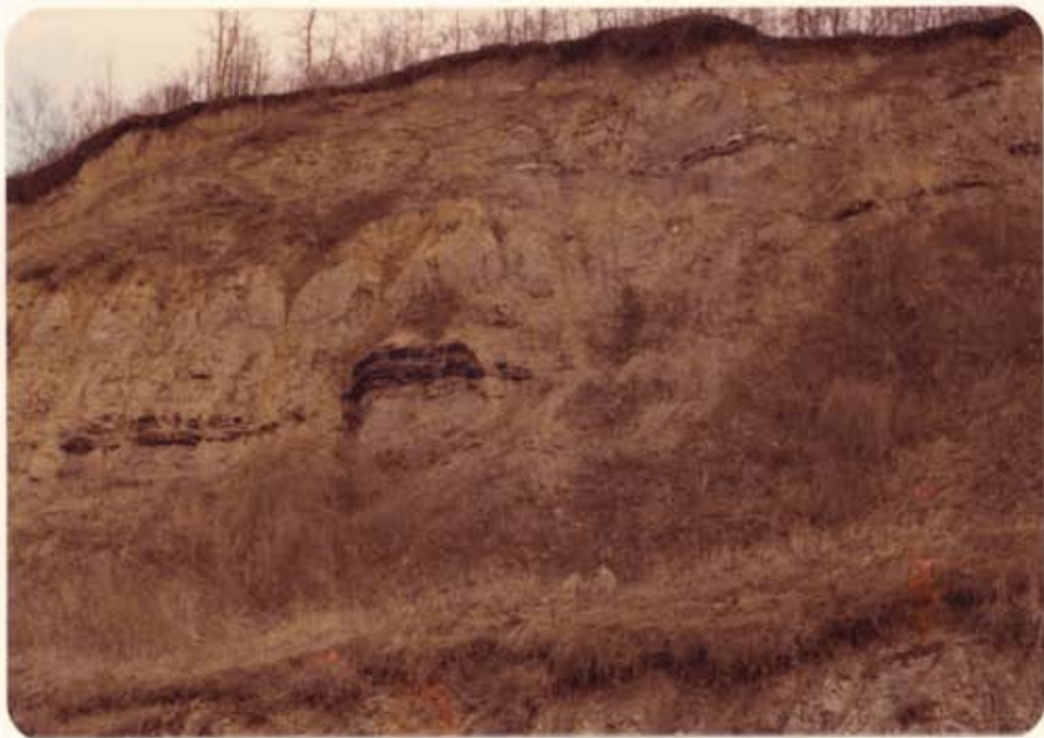
Fig. 5-3 - Dirty, oxidized coal outcrop along the B.C. Railway tracks south of Quesnel
