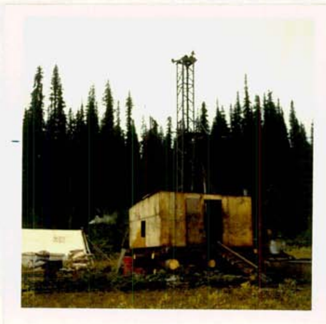
Figure 30.- Drill at diamond drill hole number three. Tent in background was used for core logging.
