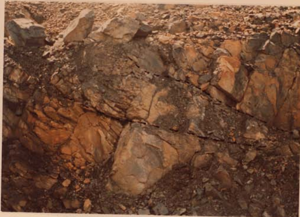
Two faults with not so noticeable displacement. Could be 5 cm or 5 m displacement.
