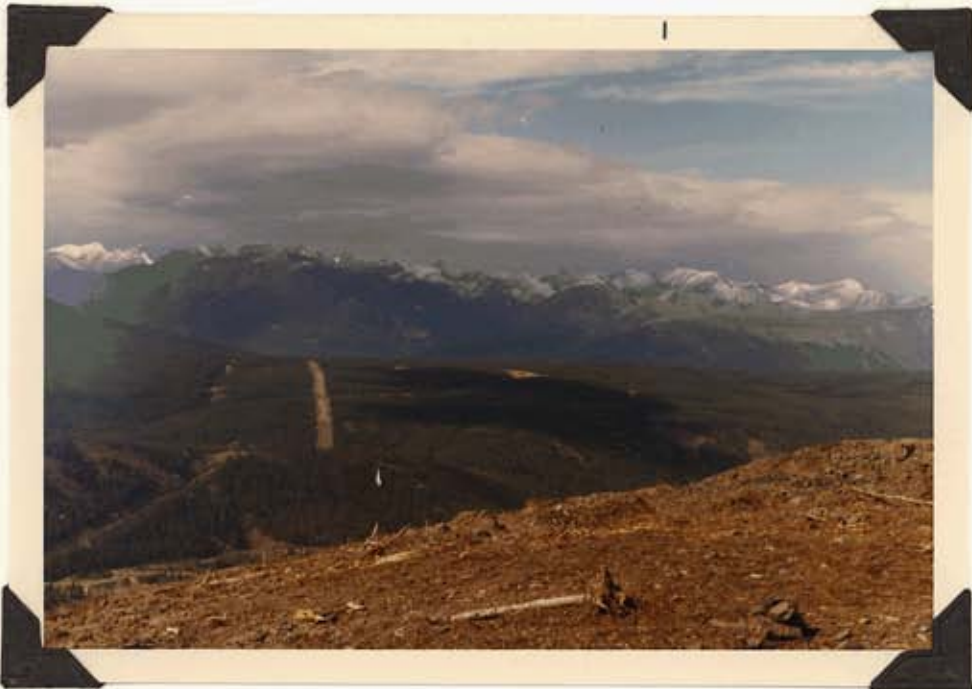
PLATE 19 - MAIN HAUL ROAD TO EAGLE MOUNTAIN PITS UNDER CONSTRUCTION.
