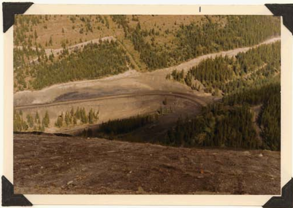
PLATE 18 - LOOKING DOWN FROM EAGLE MOUNTAIN INTO CLODE CREEK, SHOWING THE 80-FOOT WIDE MAIN HAUL ROAD.
