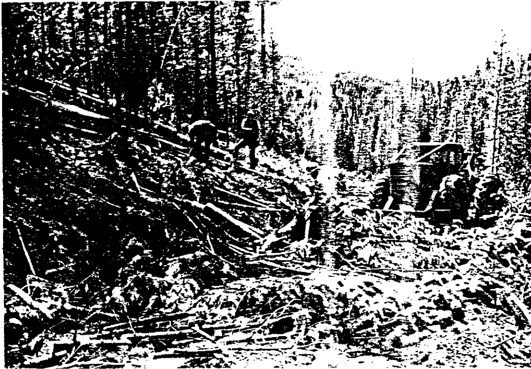
Figure 2 - Prelogging of an exploration road.
