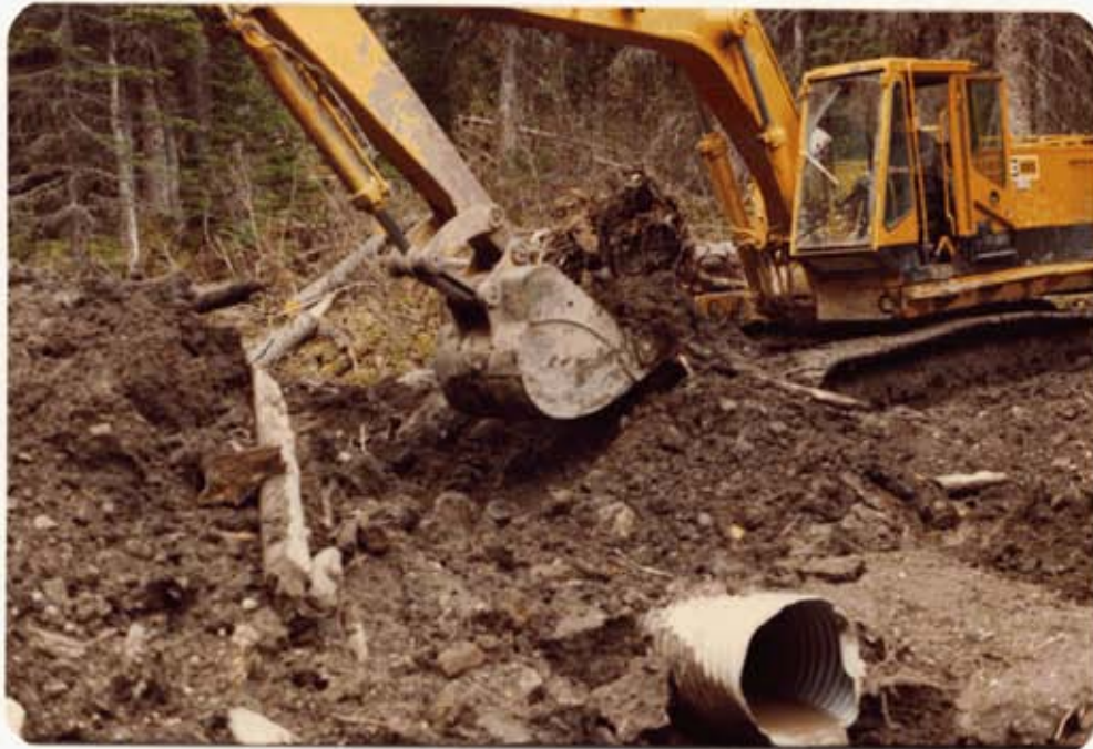
FIG. 2 CAT 225 BACKHOE REMOVING CULVERT FROM AN ABANDONED SECTION OF ROAD
