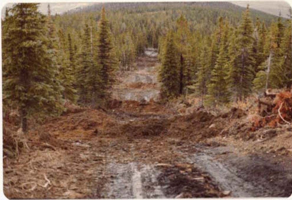
FIG. 3 EROSION BARS ON A NEWLY SEEDED SECTION OF THE ALPINE SPUR, DUKE MOUNTAIN
