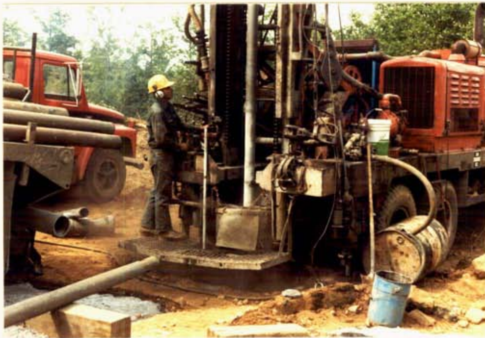
PLATE III. - Rock drilling with downhole percussion hammer.
