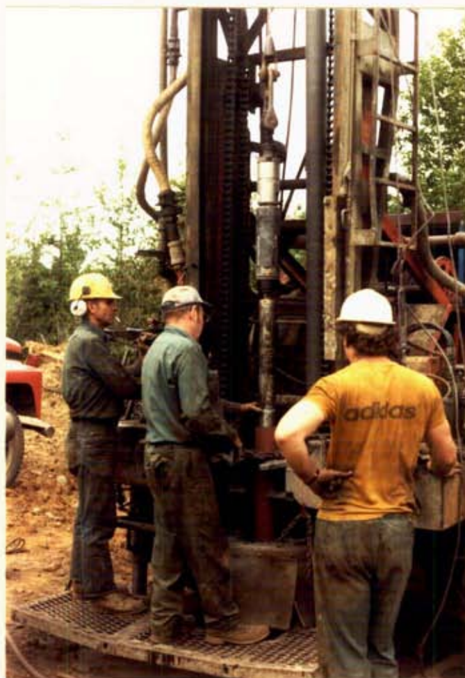
PLATE IV. - Core retrieval operations, Hole HL-84-05C.
