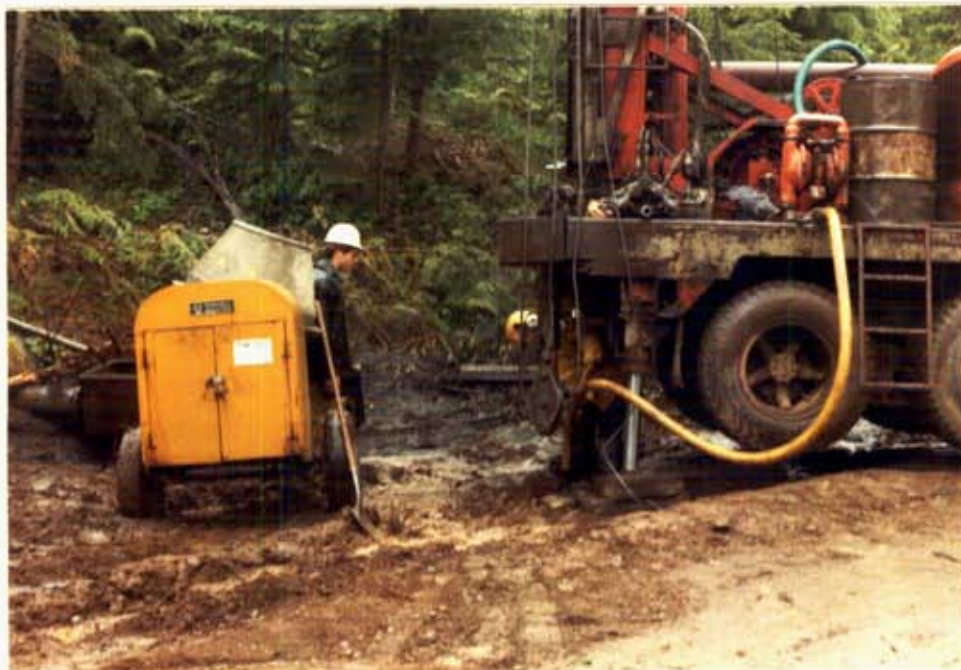
PLATE XIV. - Cementing and abandonment operations.
