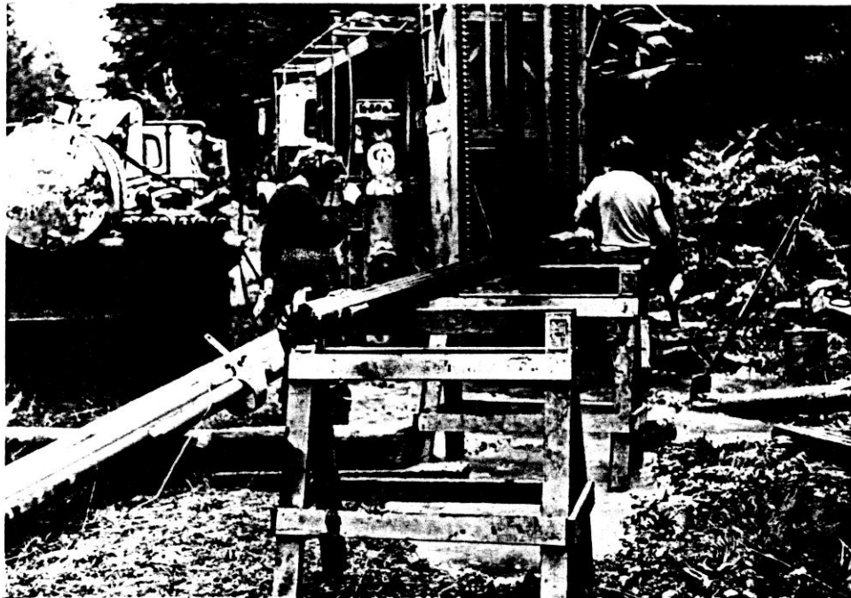
PLATE II: Retrieval of Core Barrel Upon Completion of One 10 Foot Run.
