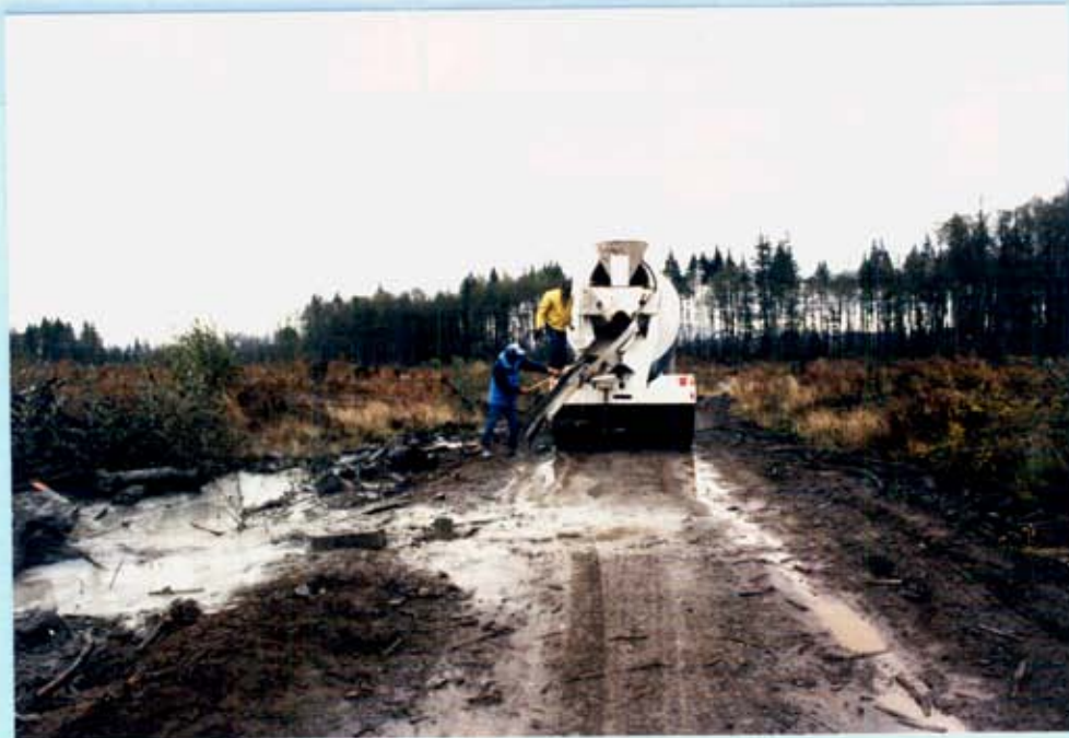
CEMENTING DRILL HOLE 88-08 ON B.C. FOREST PRODUCTS LOGGING ROAD.
