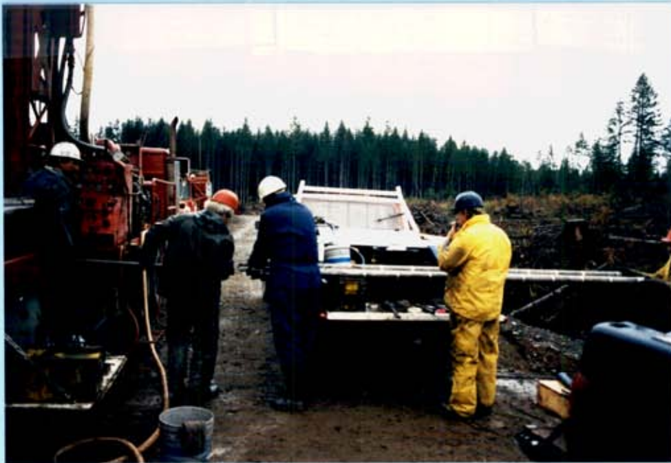
PREPARING TO PUT SPLIT TUBE CORE BARREL BACK IN HOLE 88-05
