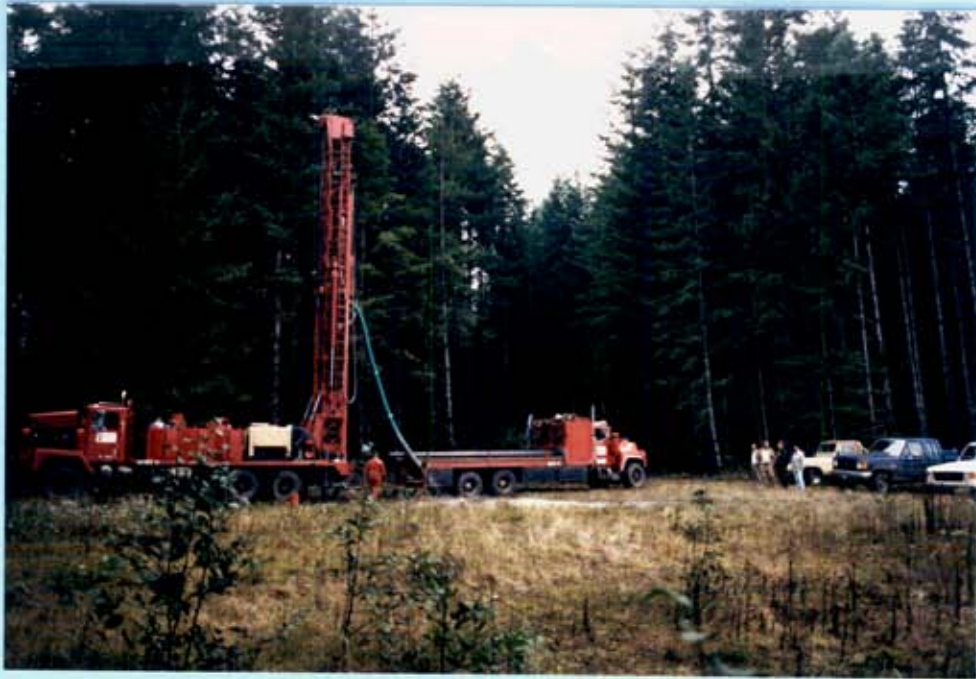
SETTING CASING ON DRILL HOLE 88-11
