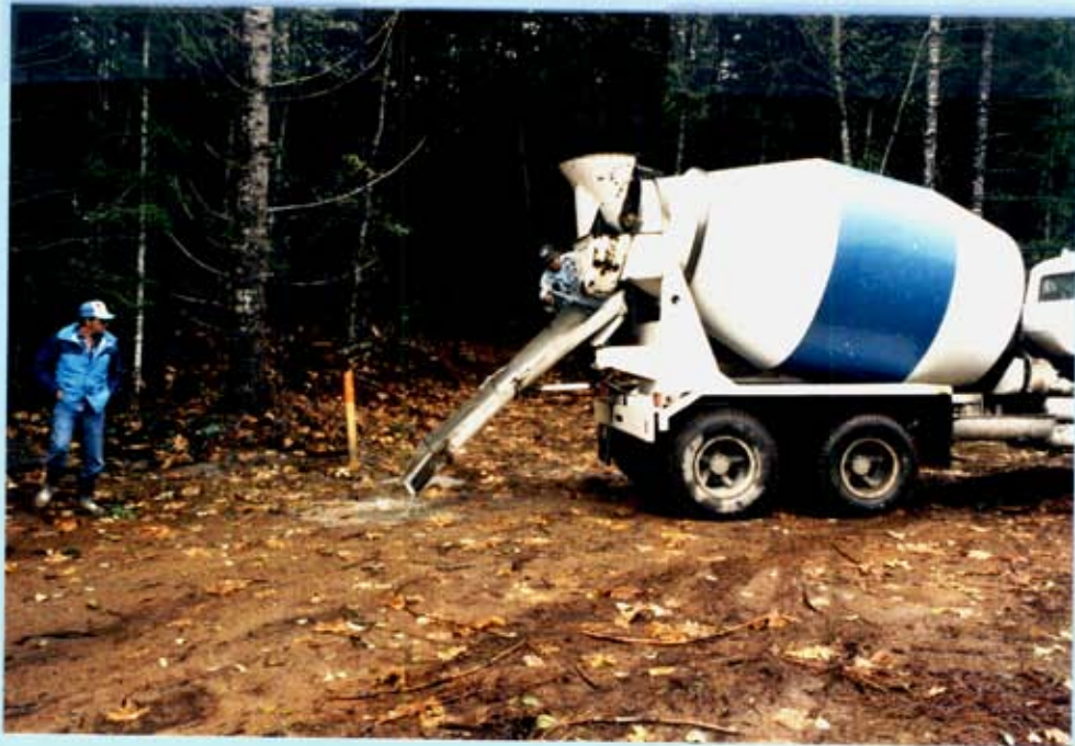
CEMENTING DRILL HOLE 88-09 ON B.C. HYDRO RIGHT-OF-WAY
