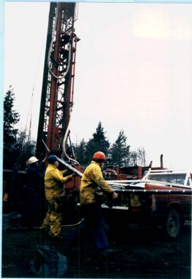
PULLING WIRELINE CORE BARREL FROM HOLE 88-05
