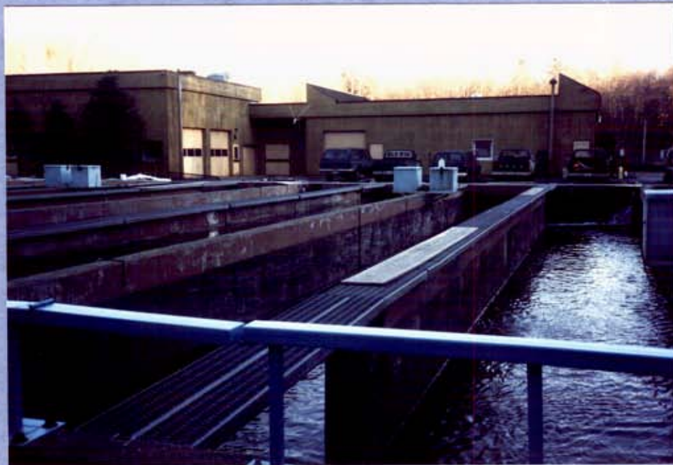
SALMON HATCHERY NORTH OF MINING BLOCK A-B AND NOT AFFECTED BY MINING ACTIVITY.
