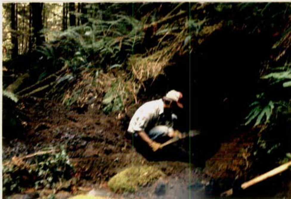
PLATE VI. - Trenching work, main coal zone on creek northwest of Log Dump.
