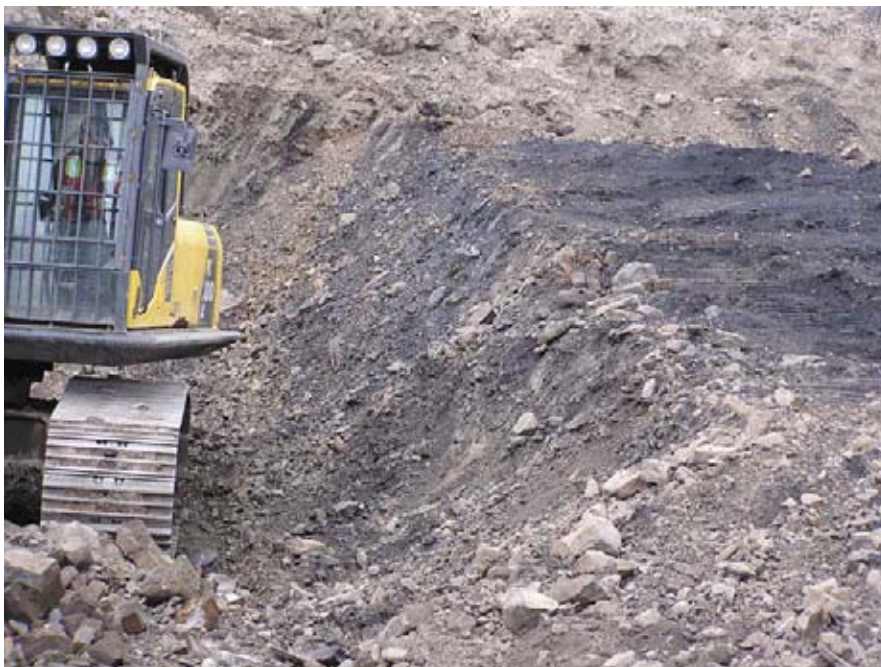
Photo 5-2 Exposing Seam D along ridge line C2.
