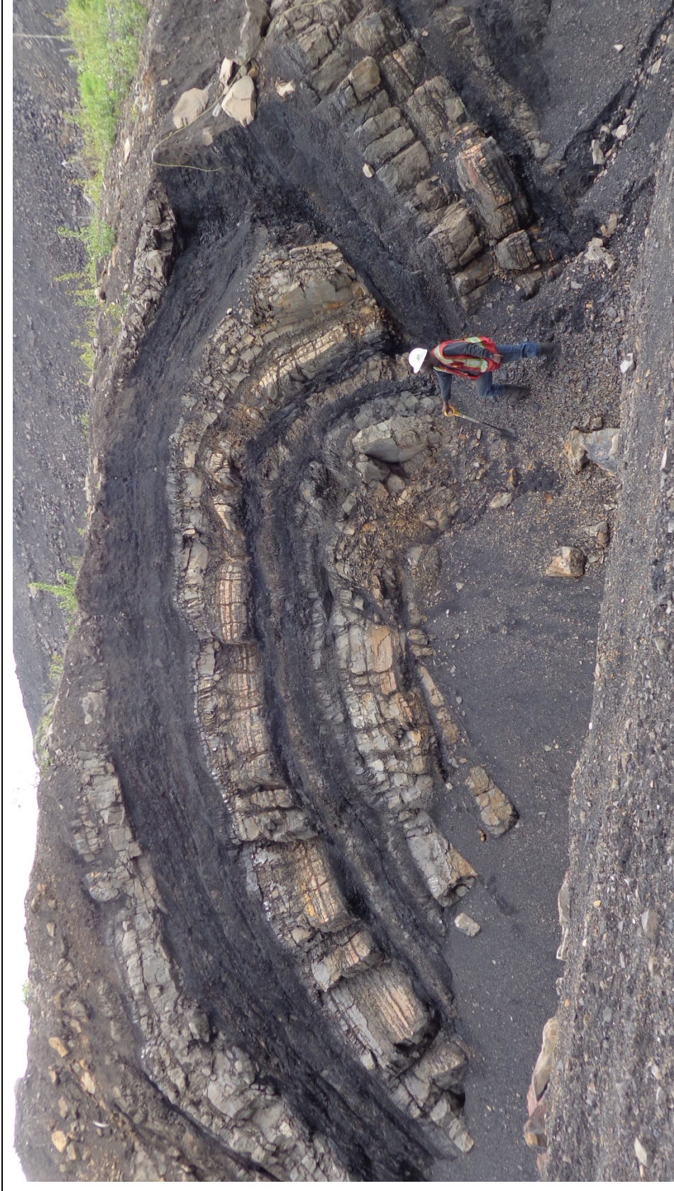
Plate 4-1: Marker A coal zone, warped into an asymmetric anticline overlying a bedding-parallel thrust fault. View is north-westward from an access road to Brule Mine's water-handling site SP-2. To the left, the overthrust rocks regain regional southwestward dip. Marker A is characteristically a doublet of coals, here mostly represented by rooted, variably-carbonaceous to coaly mudstones and impure 'dirty' coals. Colliery geologist Francis Eshun P.Geo. is the scale. [image RC1013/13]
