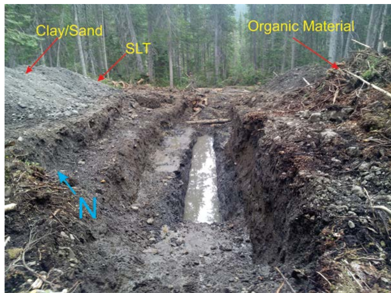
Figure 1: Trench site AC-GH-TR-03 prior to water being pumped out.
