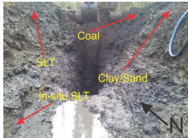
Figure 1: Overview of trench showing removed material locations.
