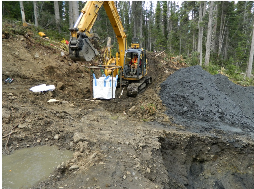
Figure 8: Apparatus used to fill one tonne ore bags with coal.
