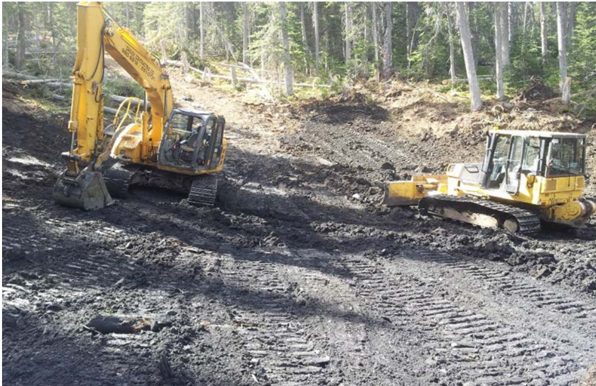
Figure 10: The trench site after the trench was filled and unconsolidated material partially spread over trench site.
