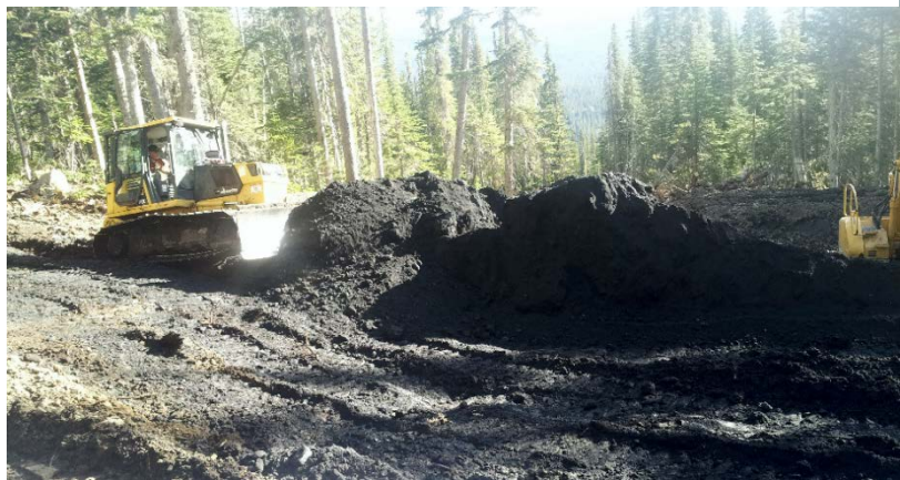
Figure 9: Operator back-filling coal into trench to start the reclamation process.
