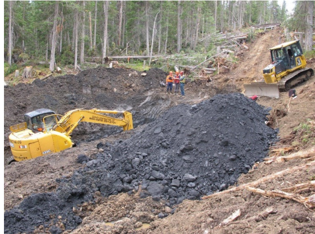
Figure 4: Overview of coal stockpile midway through trenching.
