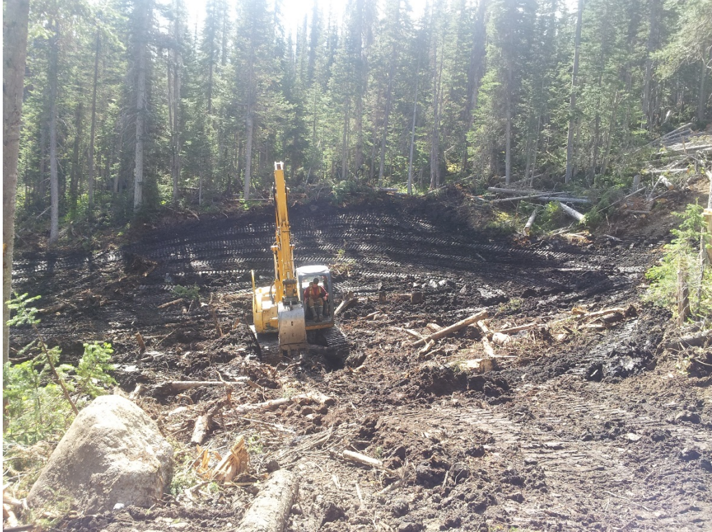
Figure 11: Operator beginning to spread the organic material over the trench site.
