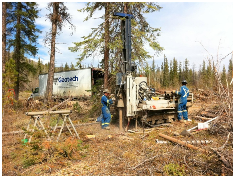
Plate 3. Drilling monitoring well MW-H22.
