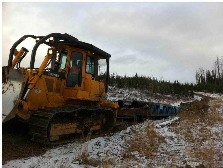
Plate 3. Road improvements and bridge install.
