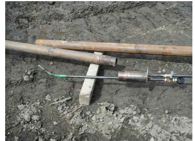
Photo 4: Photo showing the length of the short 19 mm diameter steel rod below the threaded HQ top cap. The photo shows the short 19 mm diameter pipe extends some distance (approximately 0.6 m) below the HQ top cap. The bottom of the short 19 mm diameter steel rod has a flexible polyethylene tube affixed to its base. The purpose of the flexible polyethylene tube is to prevent an air-lock from occurring within the short 19 mm diameter tube (dedicated to measuring water pressure).
