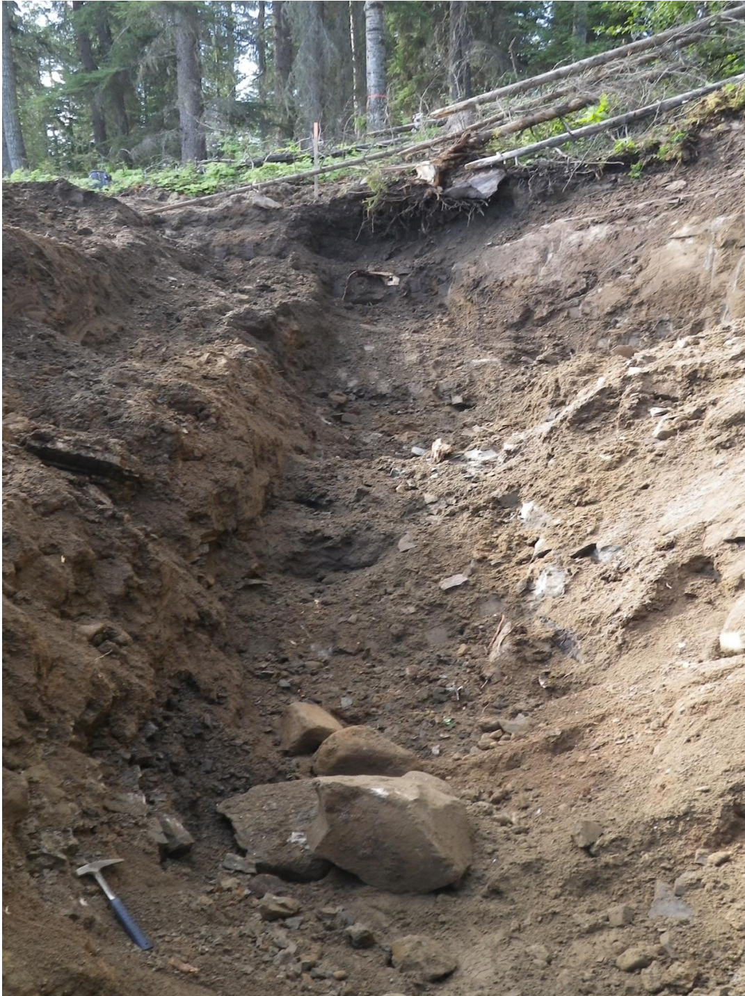
TP12-05 Photo 2 (Looking south)
