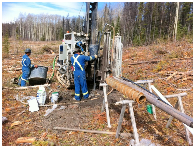
Plate 2. Drilling monitoring well MW-H19.
