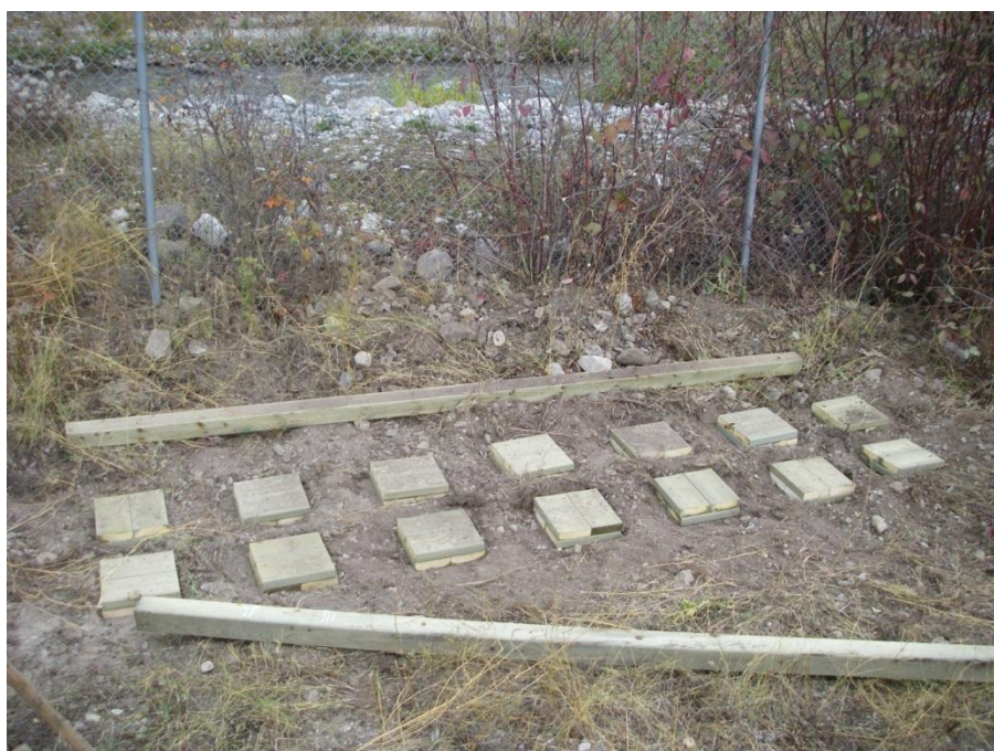
Figure 2: Foundation Establishment and Footing Placement
