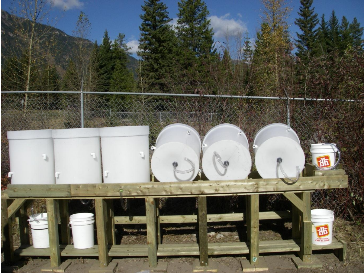
Figure 6: Installing Field Cell Fixtures and Plumbing
