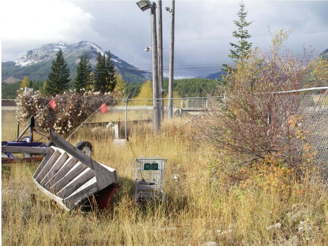
Figure 1. Kinetic Field Cell Site Location Prior to Construction – Race Trac Compound, Elkford, BC.
