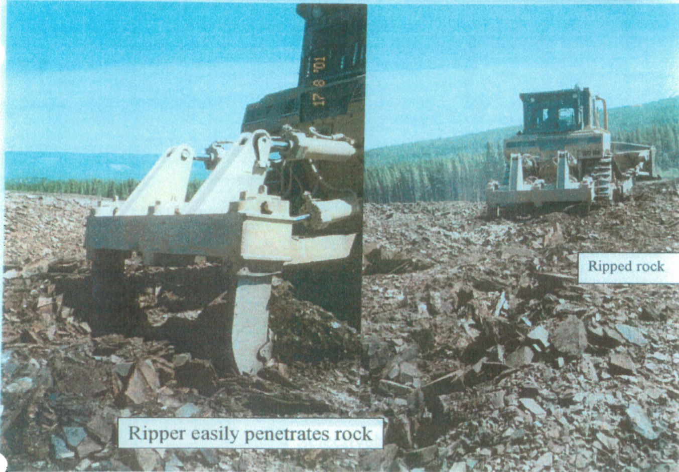
Ripping and Dozing Waste Rock to Expose Coal –August 17,2001
