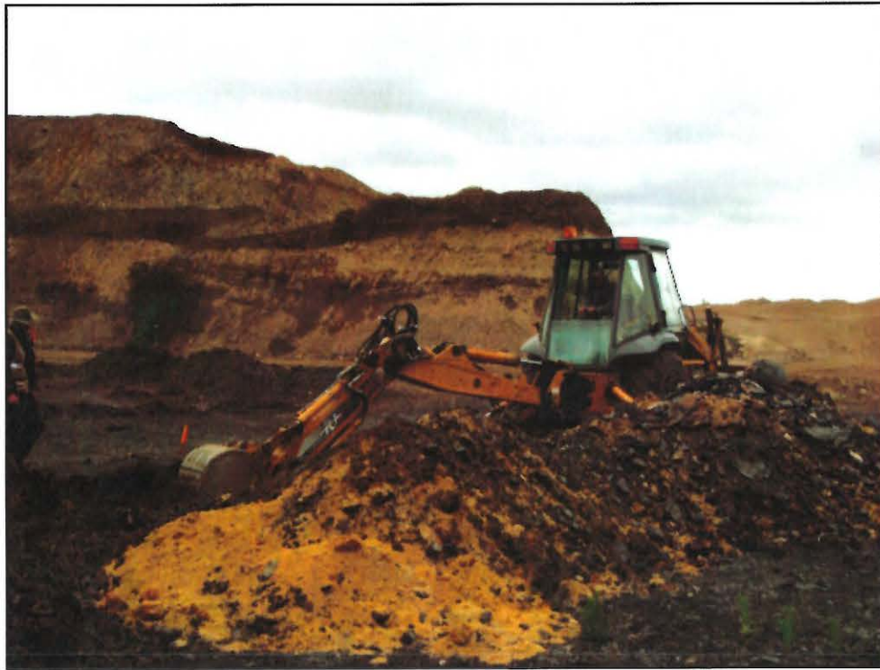
Photo 5: Bentonite extracted during 2009 trenching activity.
