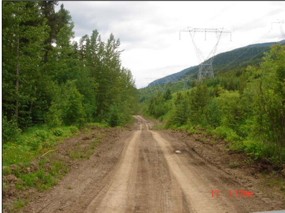
Photo 5: Example of pre-existing access (very wide) that was re-opened. Note the utilized width was kept to a minimum.
