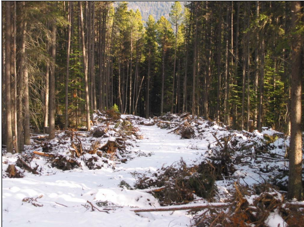
Photo 26: Reclaimed trail access showing roll backs
