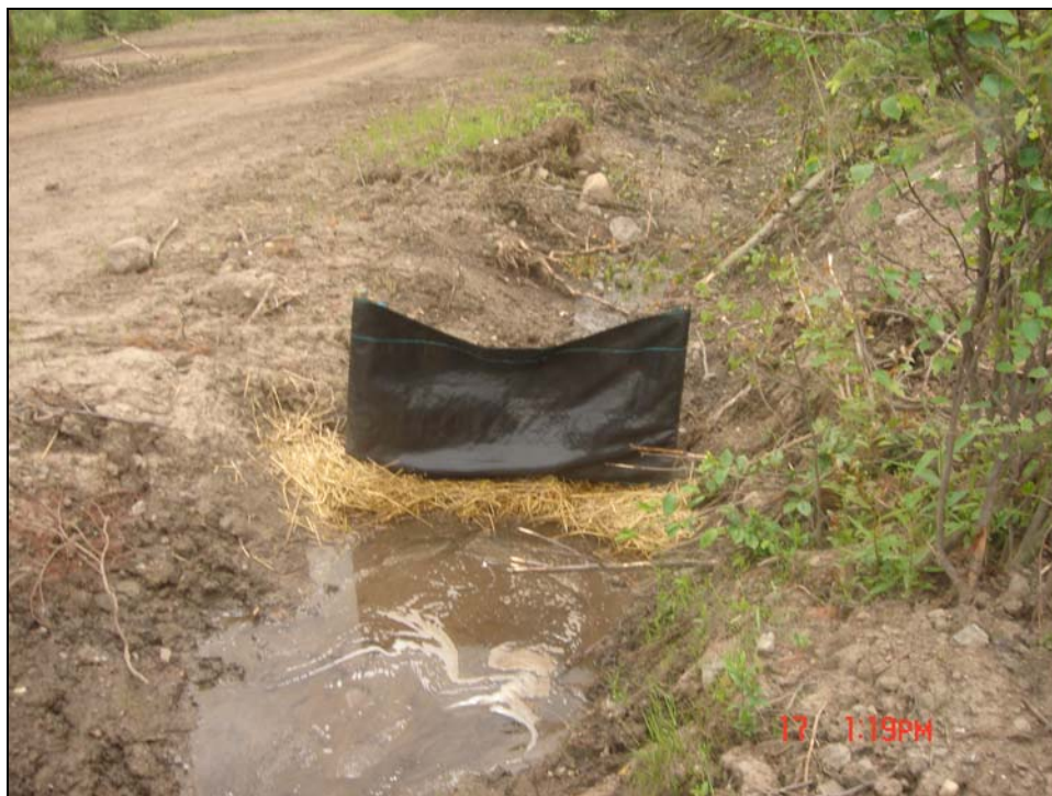
Photo 6: Example of erosion control for roads
