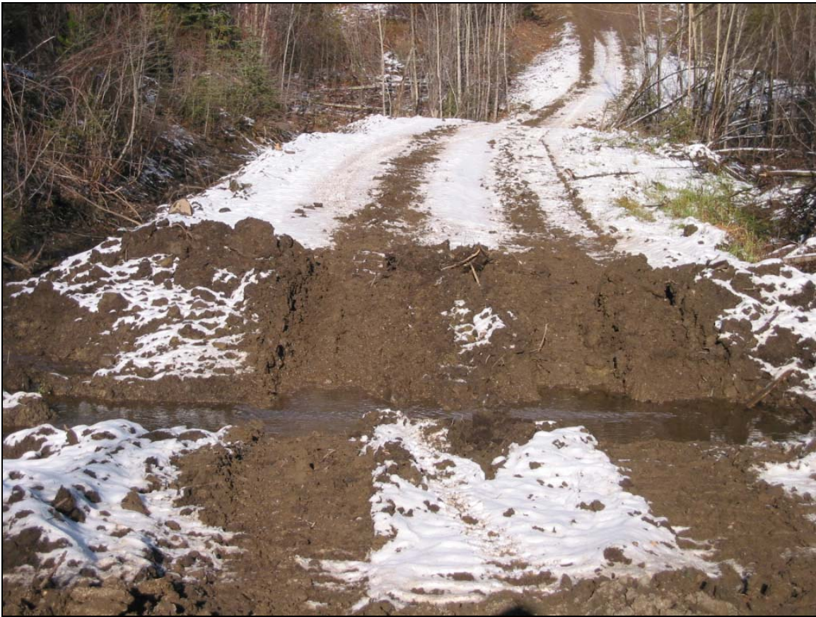
Photo 25: Cross ditching for road deactivation
