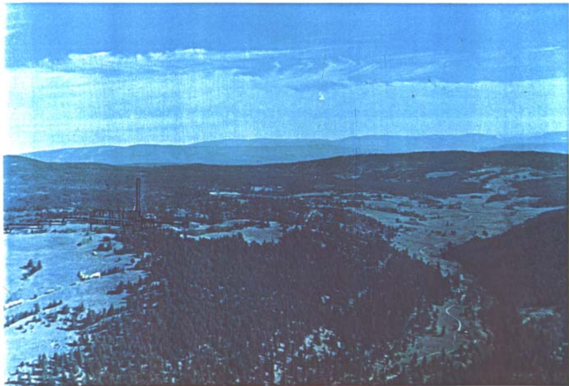
VIEW OF POWER PLANT SITE FROM THE EAST
