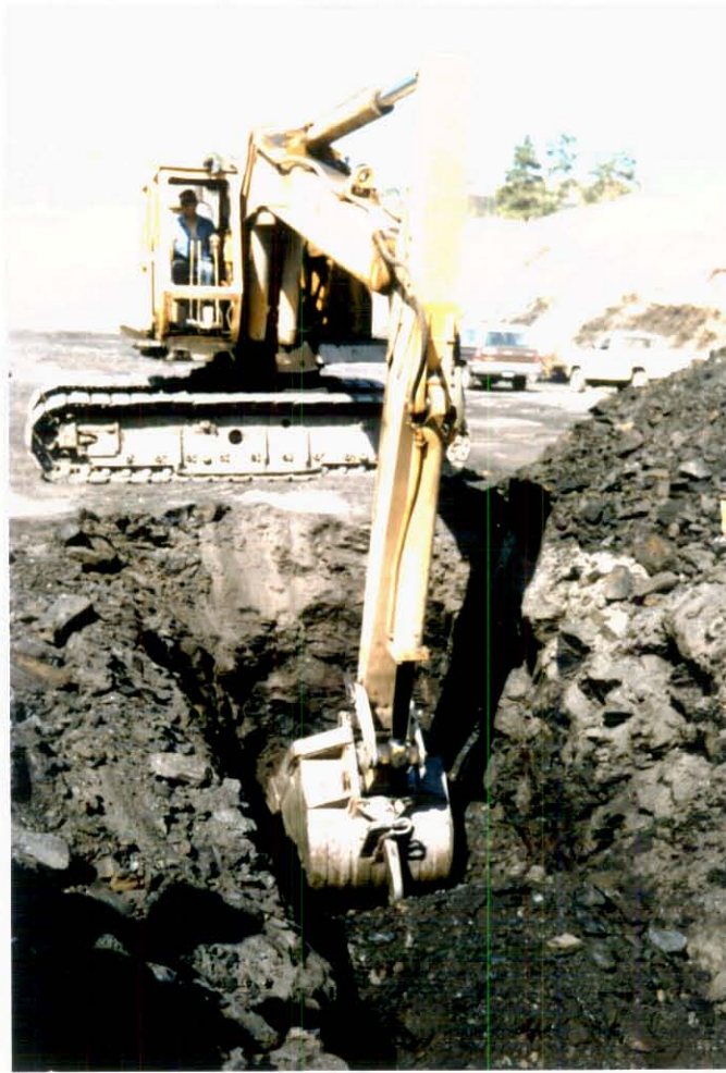
Photo 7: Excavating the 2 m x 2 m sample cut.
