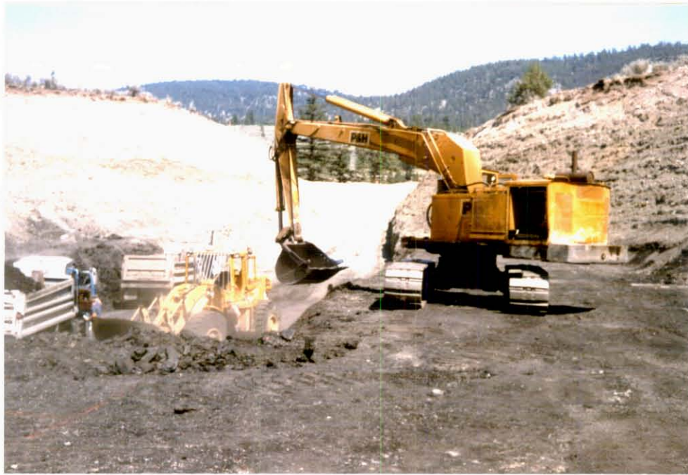
Photo 3: East end ramp completed - Starting the coal cut - P&H 418 hydraulic excavator, 966 loader, two 12-yard dump trucks.
