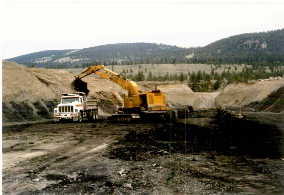
Photo 6: Backhoe loading the dump trucks from on top.
