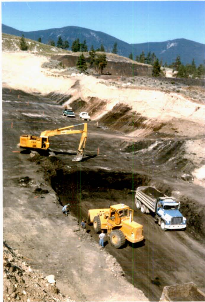
Photo 5: Front end loader loading trucks in the slot.
