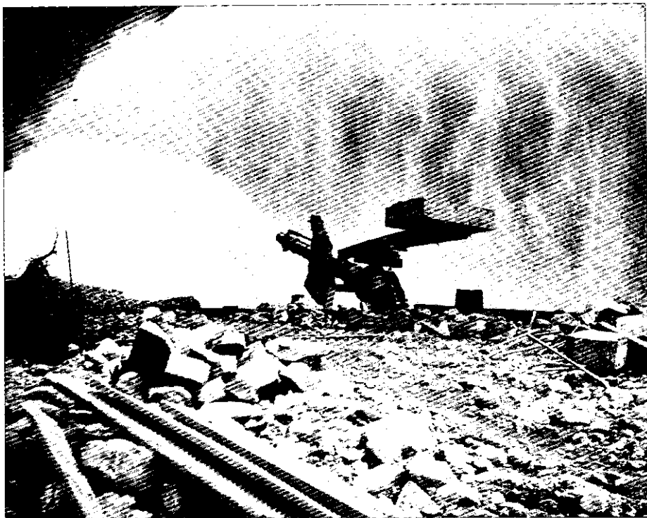
SIX INCH MONITOR IN CARIBOO MINE, NEAR QUESNELLE FORKS.
