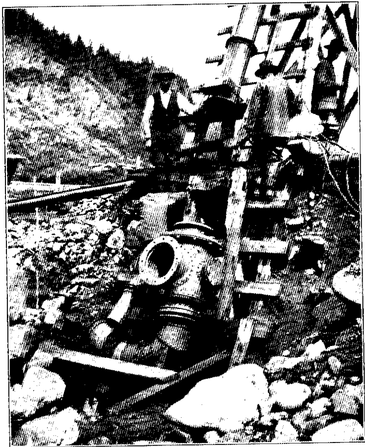
SETTING UP HYDRAULIC ELEVATOR.
