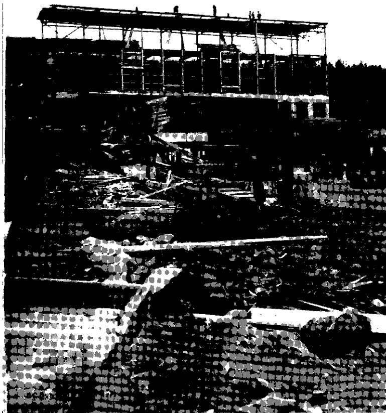
Sullivan Mine, Kimberley, Fort Steele M.D.—New Concentrator under Construction.
