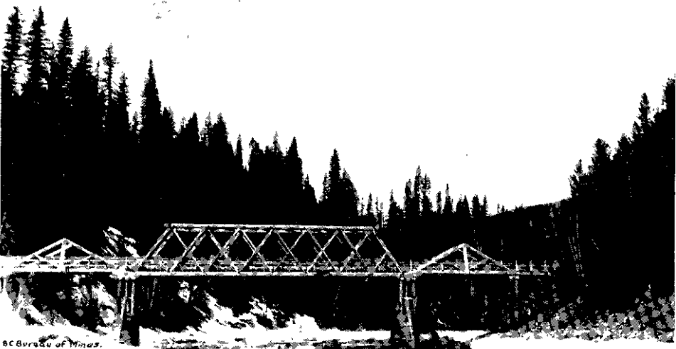
Spanish Creek Bridge, Quesnel M.D.
