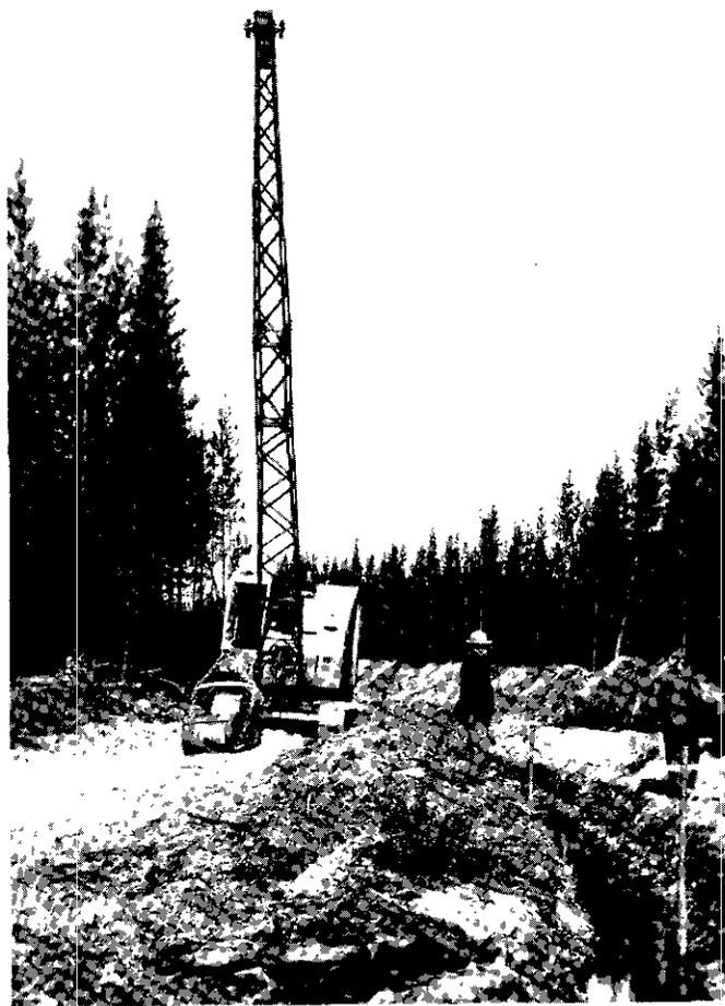
Ditch-construction using boom drag-line, Germansen River. operation of
