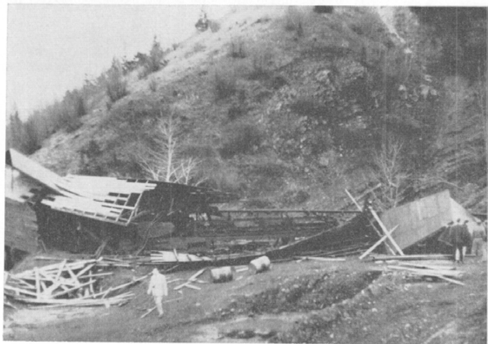
Plate XIb. Balmer North mine. Portal of No. 1 tunnel showing wreckage between portal and truck-loading bin.
