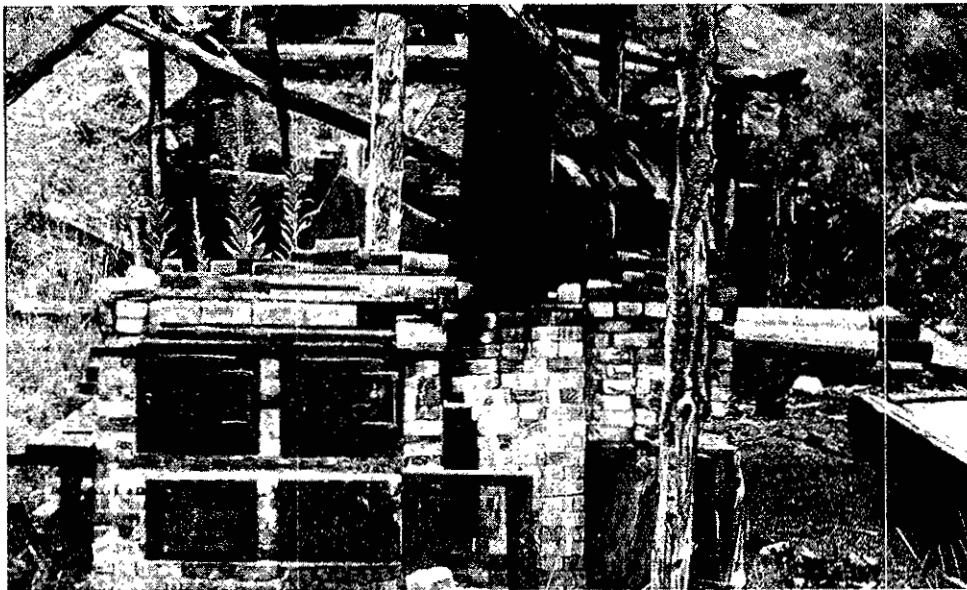
B. Small D-retort at Copper Creek cinnabar property.
