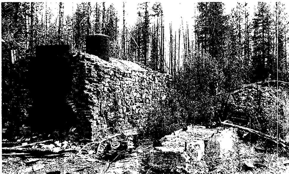
Minnie-ha-ha boiler and hoist foundation, shaft in right background.
