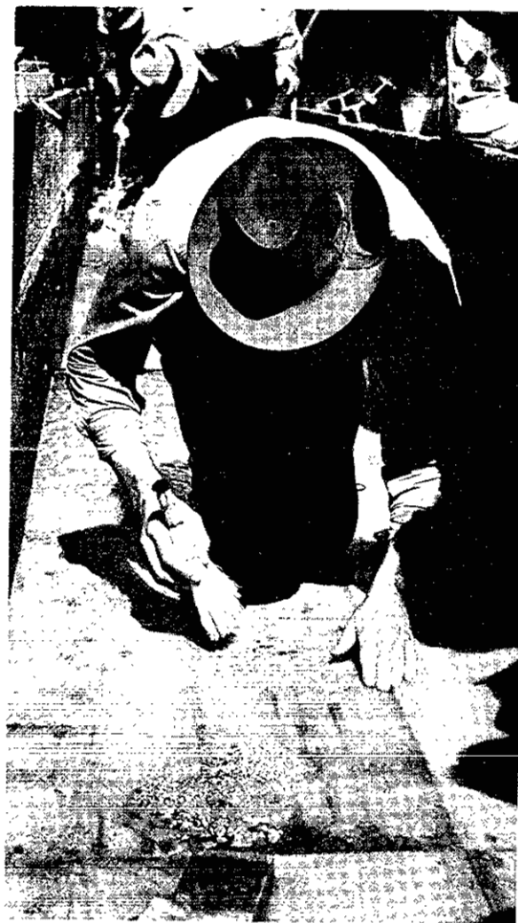
Plate XV B. Cleaning up the gold in the bottom of a sluice-box to remove as much black sand as possible before scooping up the gold into a pan.
