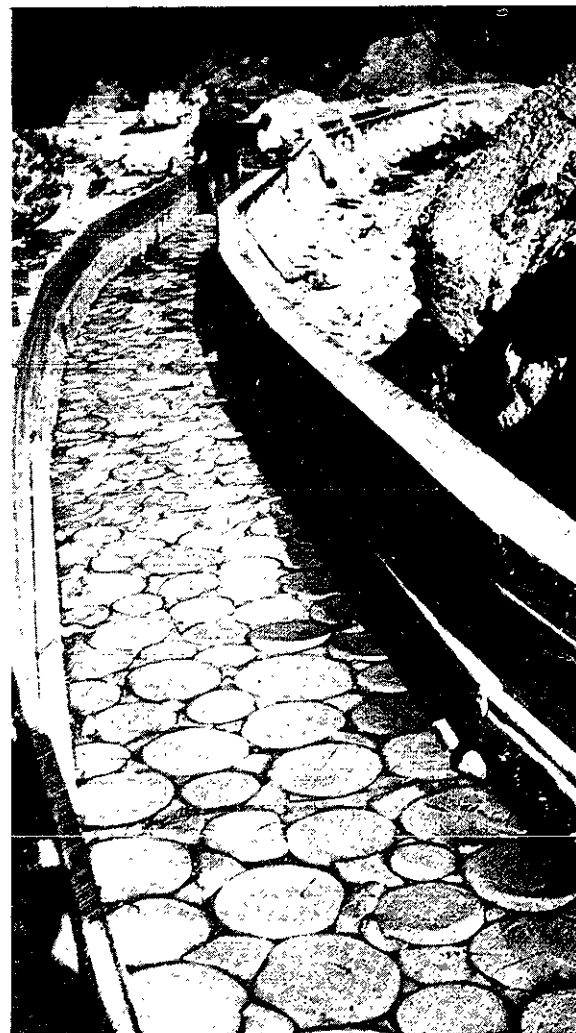
Plate IX B. A large sluice-box paved with wood blocks wedged together by blocks in the interstices. A safety stick is nailed across at the end of each 12-foot box.
