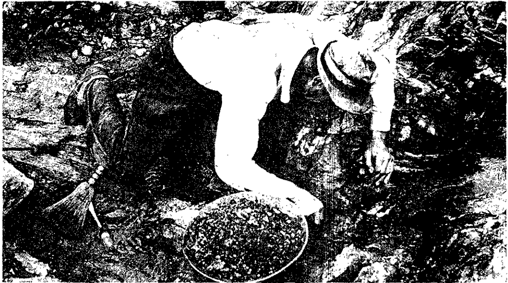
Plate XVI A. Cleaning bedrock by hand. At Germansen Ventures the bedrock is hard and irregular so that it is impossible to clean it adequately with the giant. One man is continuously employed cleaning out all the cracks by hand.
