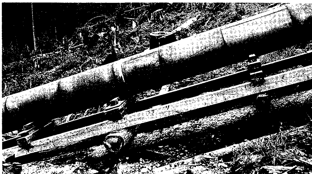
Plate IV B. Part of the main 30-inch section of the Bullion pipe-line showing the foundation supports.
