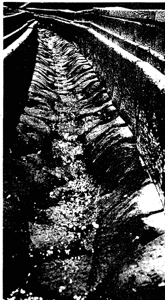
Plate X B. A 30-inch sluice-flume showing a central groove worn in the wood block riffles after considerable service.
