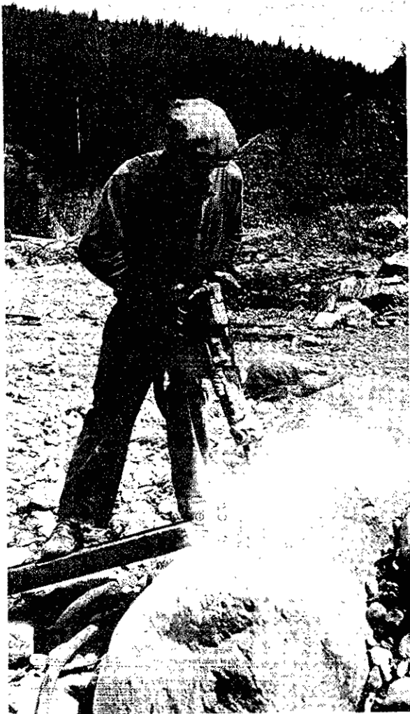
Plate XIV A. Drilling a large boulder with a jack-hammer in the hydraulic pit at Spanish Creek, B. C.
