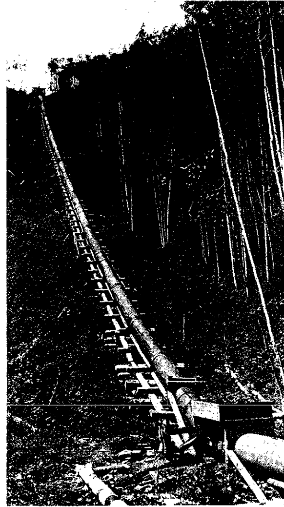
Plate III B. A section of 24-inch pipe-line leading from the penstock at Cariboo Cottonwood Placers Ltd. This is a well-laid pipe-line; notice the supporting cribbing for the pipe and the bracing at the change in grade of the pipe.
