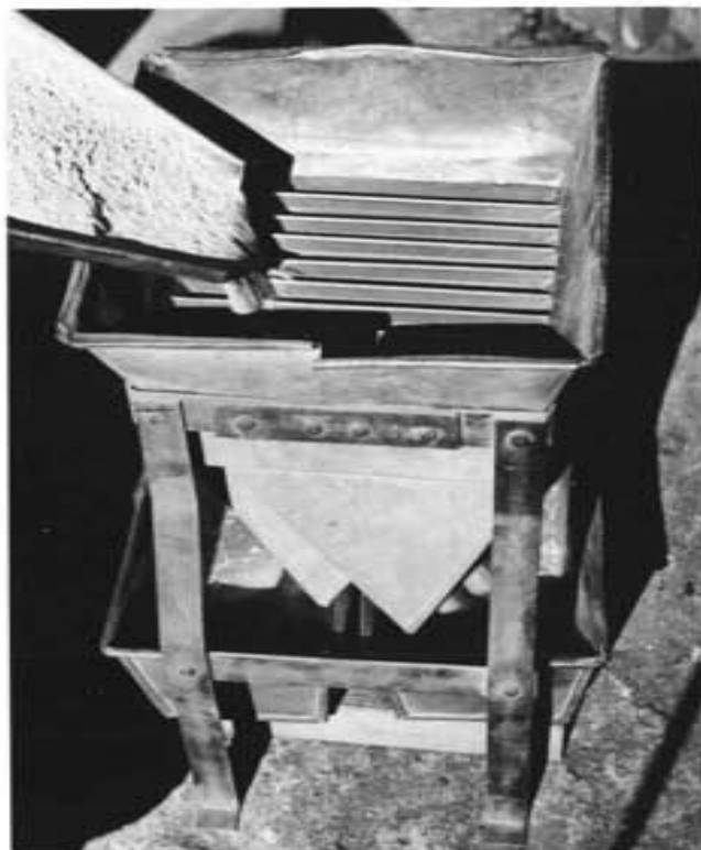
B.—After crushing the sample it is sampled in this Jones riffle, the falling ore being split into two streams by the metal partitions shown. One-half of the sample goes to the left-hand pan, the other half to the right-hand pan. The contents of either pan may be taken for further grinding and sampling.
