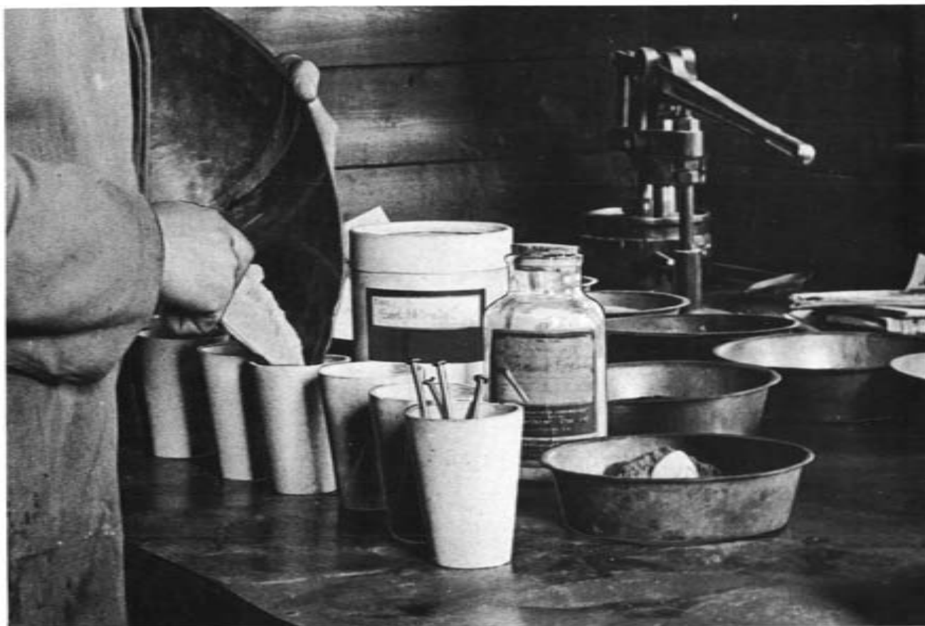
A mixture of ore and fluxes being put in a crucible for a precious metals assay.
