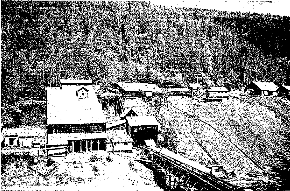
A. Whitewater concentrator and surface plant. The portal of No. 14 adit is at the left of the low building against the hillside. The trestle in the foreground carries concentrates across Kaslo Creek to the railroad.
