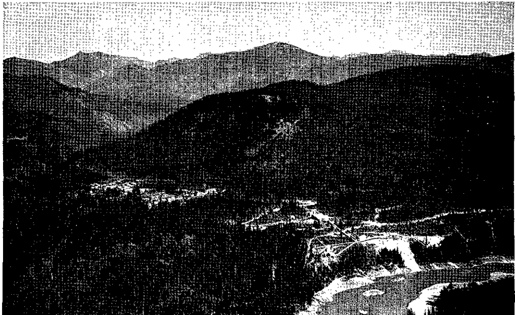
Reeves MacDonald mine, mill, and townsite looking northeast across the Pend d'Oreille River. Valley of the Salmo River left centre, Mount Waldie (left), and Lost Mountain (centre) on the skyline.
