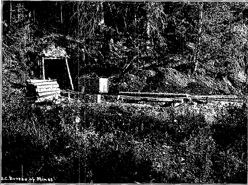
Crosscut Tunnel, No. 1 Seam—Coal Creek.
