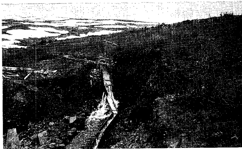
Nord Bros.' Cascade Method of Sluicing, Wright Creek.
