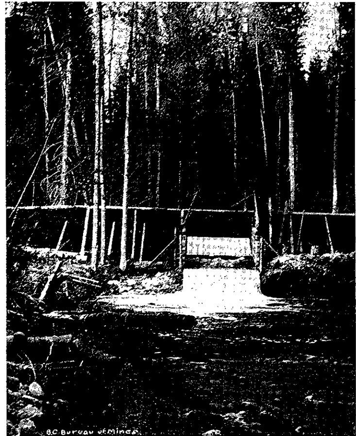
Rock Creek—Dam and Boomer for sluicing Gravels.
