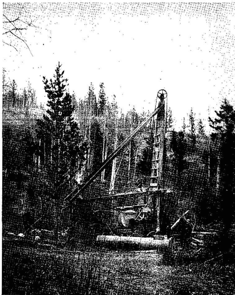
Horsefly River—Keystone-drilling of Placer-gravels.
