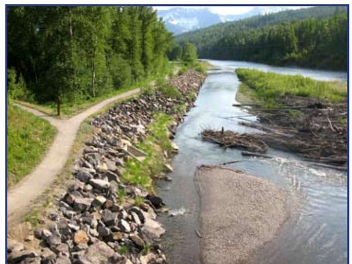
*Figure 65. Dykes built of sandstone blocks help to prevent flooding of low lying areas along the Elk River. The dykes also prevent the river channel from migrating into the town.*
