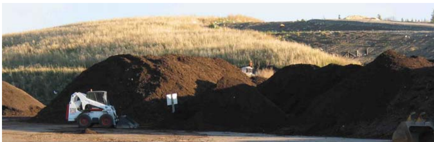
Figure 22. Compacted garbage is ready for a cover of soil. The dumped soil will be spread across the garbage to create a refuse cell. The soil-covered slope in the background is underlain by many refuse cells.
