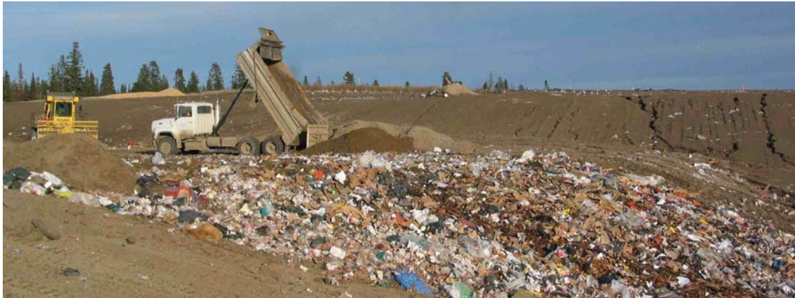
Figure 22. Compacted garbage is ready for a cover of soil. The dumped soil will be spread across the garbage to create a refuse cell. The soil-covered slope in the background is underlain by many refuse cells.
