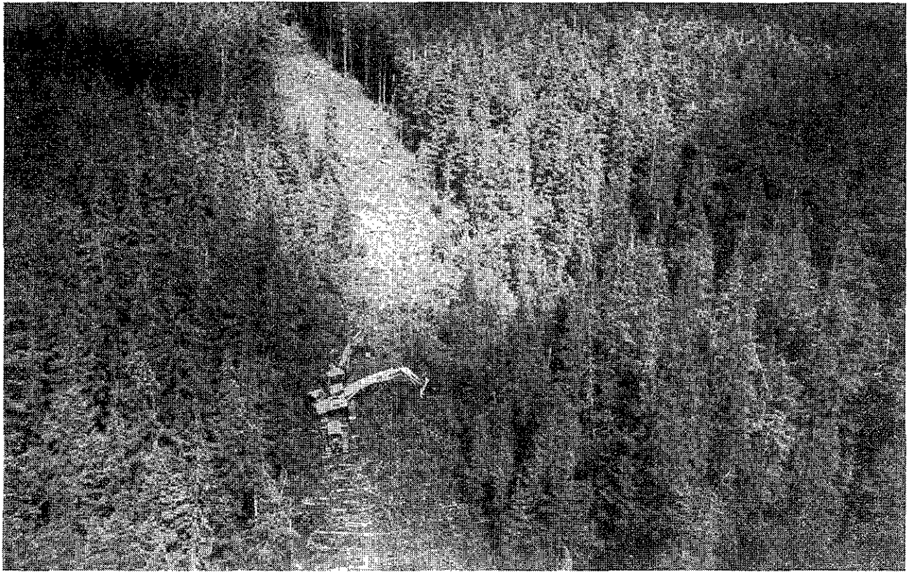
Plate A-1. Logging equipment is shown clearing the right of way on the Iskut Road. Beginning several kilometres south of Bob Quinn, the Iskut Road has been taken 37 kilometres to the west to the confluence of Volcano Creek with the Iskut River.
