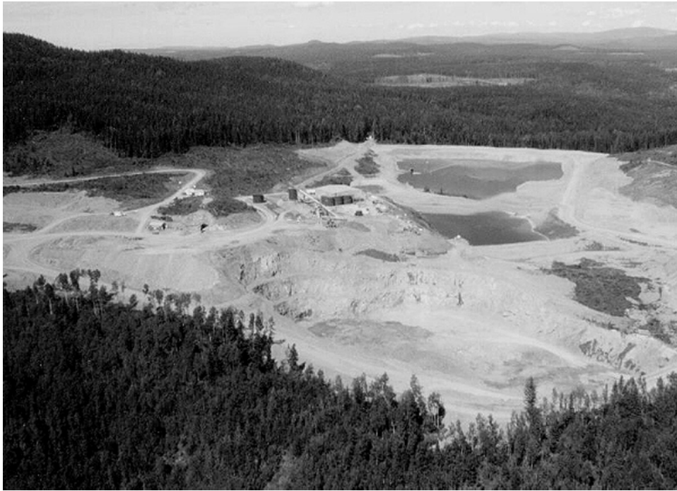
Photo 1. Looking northwesterly over the QR gold mine. The Main zone open pit is in the foreground. The carbon-in pulp cyanide leach plant and ore stockpile (centre) are flanked to the left by the Midwest zone portal, above which is situated the mine office (white building). Water storage pond and tailings dam are to the right of the mill. The West zone is off the photograph to the left or west (photograph taken by Ed Beswick, August 13, 1996).
