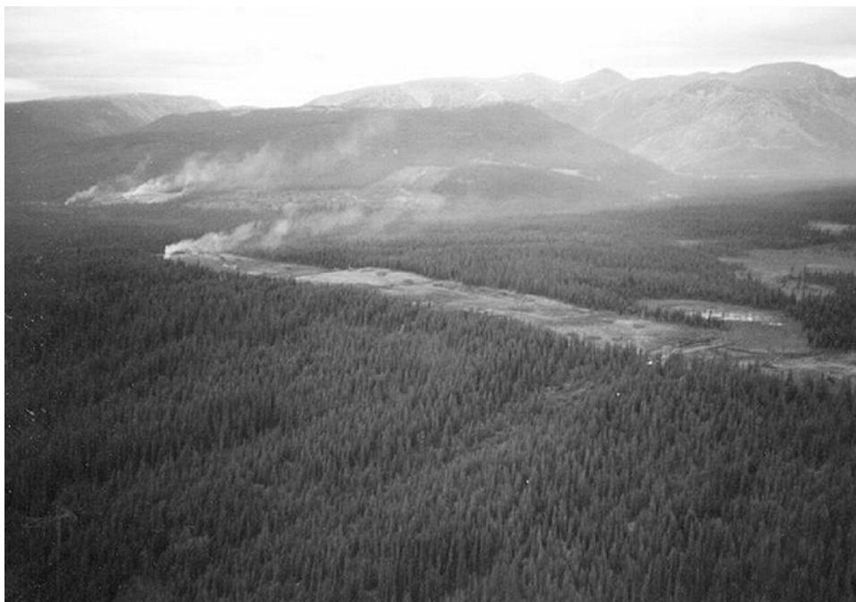
Photo 3. Looking north toward the Kemess South mine development project, July 30, 1996. The cleared area in the centre is now an operational airstrip and the cleared areas in the background, from left to right, now house the completed permanent camp, and mine and mill buildings which are under construction.
