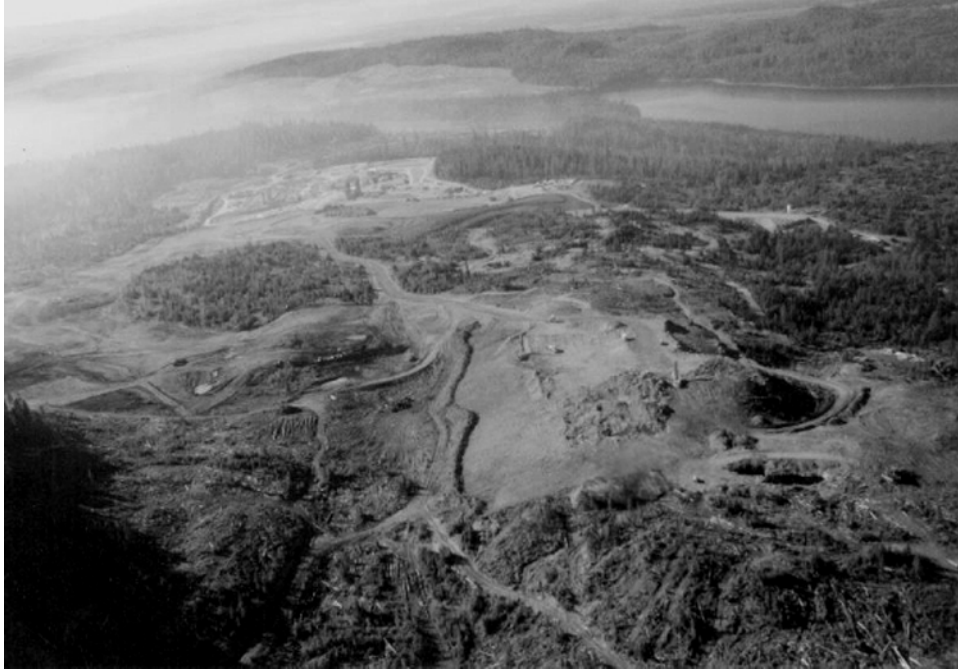
Photo 2. Looking southerly over the Mount Polley mine development with Bootjack Lake in the upper right. Rows of blast hole cuttings identify the starter pit (centre) and construction of the crusher and concentrator buildings are beginning to take shape in the upper left. Areas cleared in the middle and foreground will be part of the open pit (photograph taken by EdBeswick, August 13, 1996).
