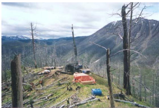
Photo 4. Drilling at Coyote Creek Property.
