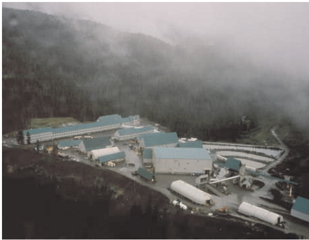
Photo 1. Eskay Creek mine surface facilities including (from left to right) living quarters, warehouse, office/mine dry, mill (largest building) and two direct-shipping ore sheds (foreground).
