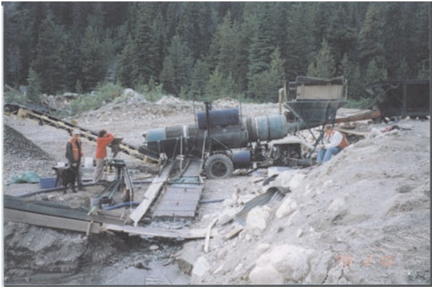
Photo 6. View of washplant and clean-up jig on McConnell Creek, V. Pogovec.
