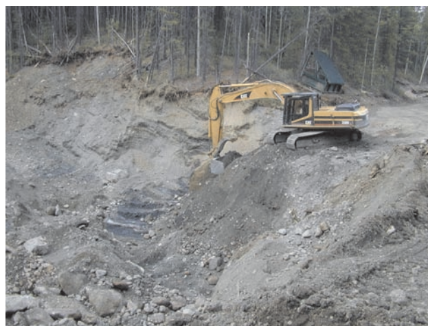
Photo 5. Excavating material from paystreak on Manson Creek, Angel Jade Mining.
