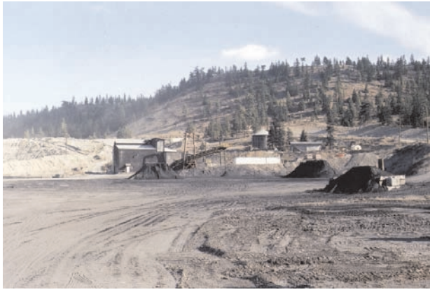
Photo 3. Processing plant and stockpiles, Craigmont magnetite tailings operation.
