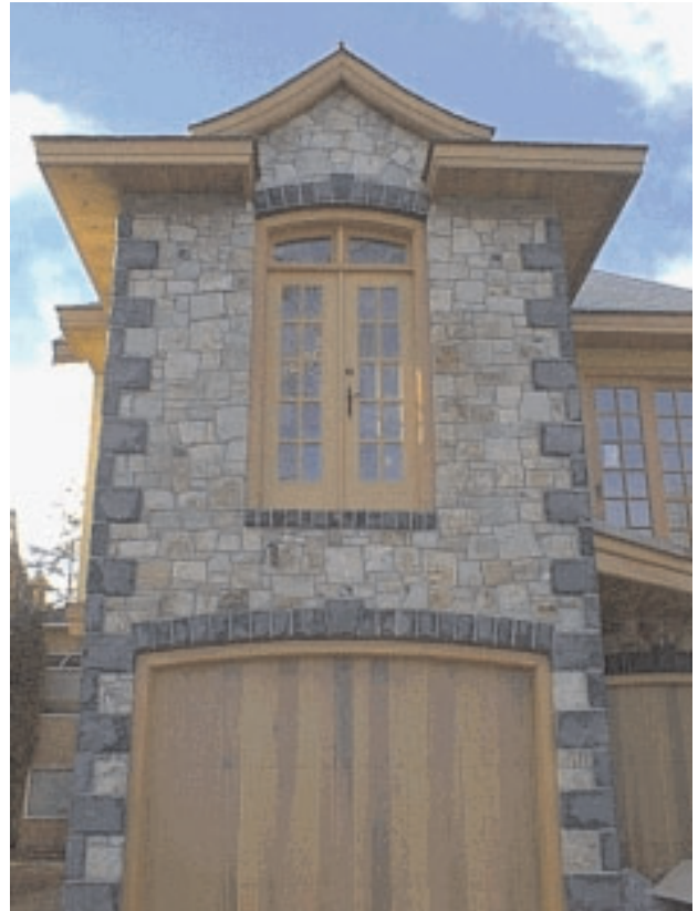
Photo 5. Home constructed using "Mountain Ash" (dacitic ash) and "Shadow Ridge" (basalt) facing stone. Photo courtesy of Kettle Valley Stone Company.
