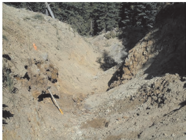
Photo 5. Trench TK99-1, Crowsnest project.
