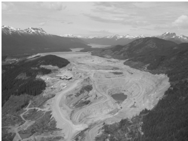
Photo 1. View west over the Huckleberry open pit mine showing Phase 2 stripping on the high wall of the East pit. The concluded Main pit and tailings pond are in the middle distance and Tahtsa Reach is in the far distance.
