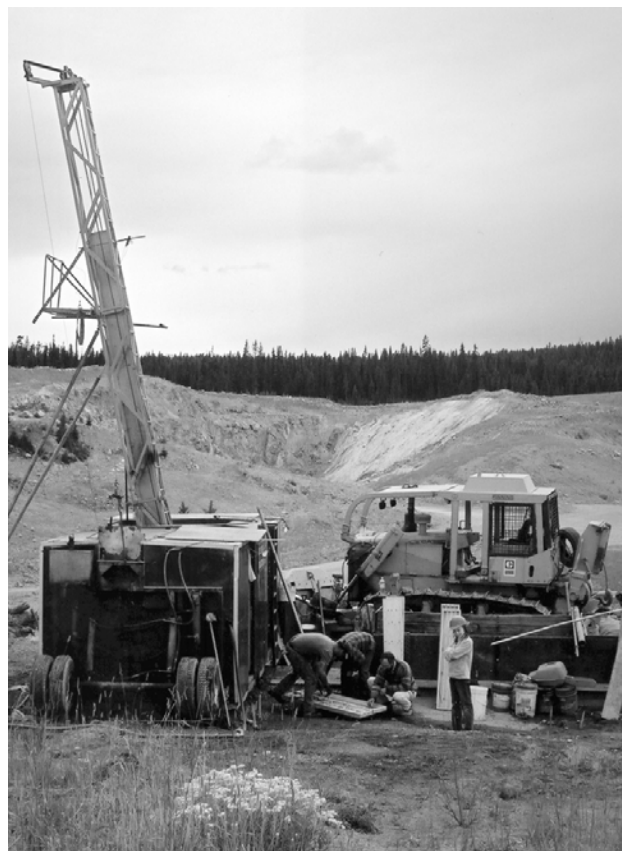
Photo 4. Drill at Elk project with Siwash North pit in background.
