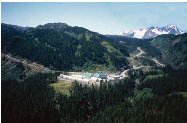
Photo 2. Looking southwesterly over the Eskay Creek gold-silver mine in northwestern British Columbia.
