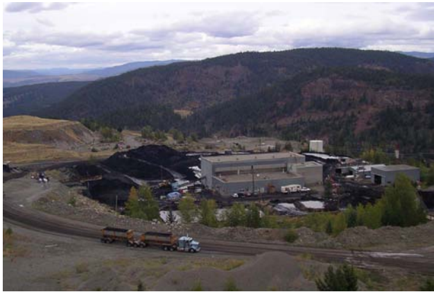
Figure 4-7. Coal wash plant of Compliance Energy Corp, located on the site of the dormant Similco copper-gold mine near Princeton.
