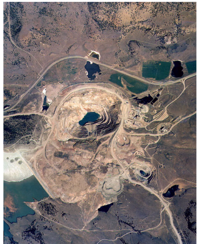
Figure 4-12. Aerial view of the Afton mine complex with the Afton pit in the centre with mill/office buildings to the east (right) and the Pothook pit to the southeast. The Afton main zone extends in a southwesterly direction from the bottom of the pit towards the tailings pond in the lower left. The Trans-Canada Highway curves around the north side of the pit. (Courtesy DRC Resources Corp)
