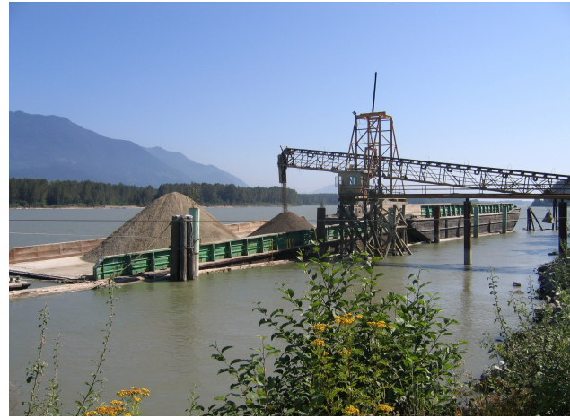
Photo 3. Cox Station quarry loadout along the Fraser River, Lower Mainland.
