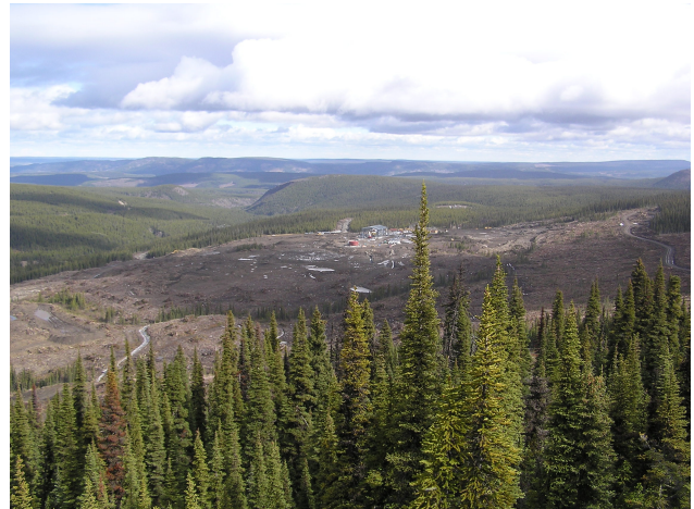
Photo 6. The Trend coal mine is scheduled for production in early 2006.
