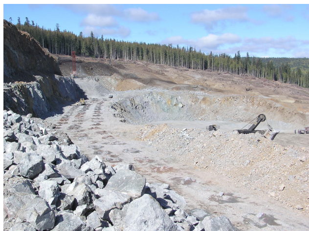
Figure 3.4. Development of the new Wight Pit, Mount Polley mine.
