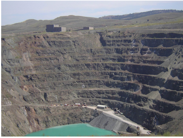
Figure 4.10. View showing the pit, portal and surface facilities at the New Afton copper-gold project of New Gold Inc.
